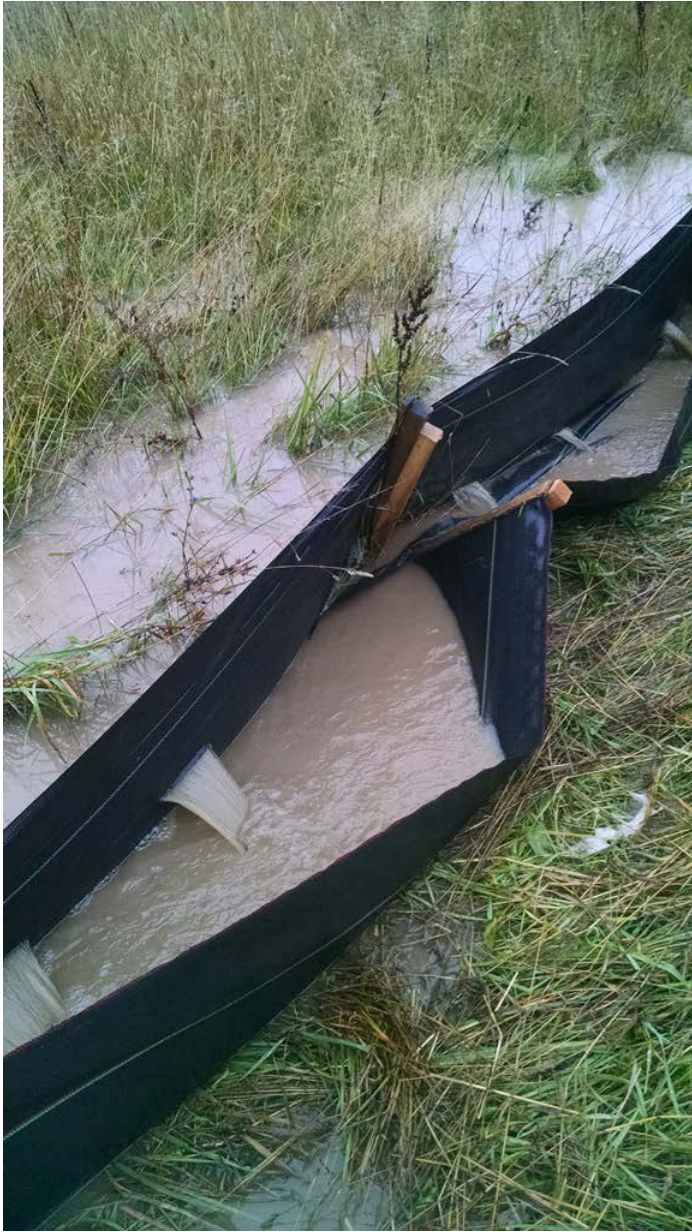
Silt fence at SE corner of VGT site
