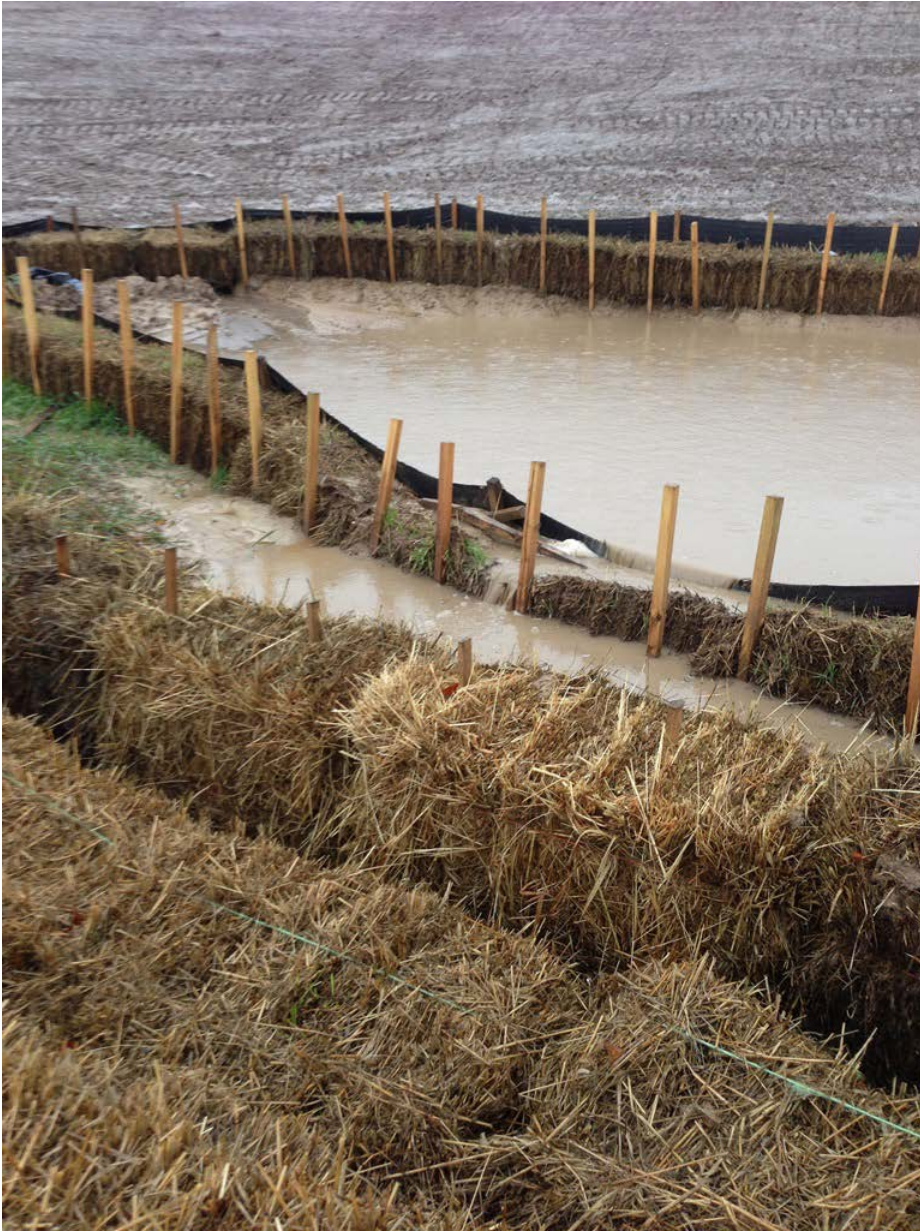
Over topping silt fence and first straw at wetland area
