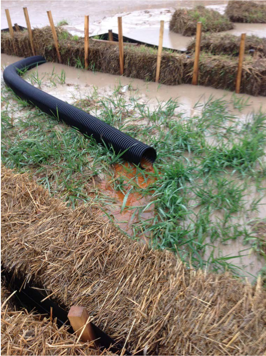
Containment at wetland
