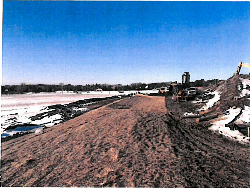
Photograph No. 15: Surface Berm and Swale Construction – Matting Placement and Swale Outlet (1/20/15)
