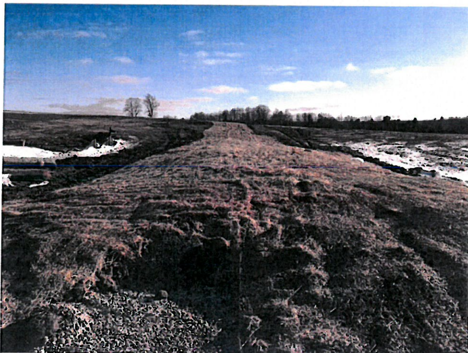
Photograph No. 13: Surface Berm Construction – Matting Placement and Swale Outlet (1/20/15)
