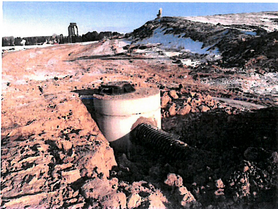
Photograph No. 11: Surface Swale Inlet Structure Construction (1/20/15)
