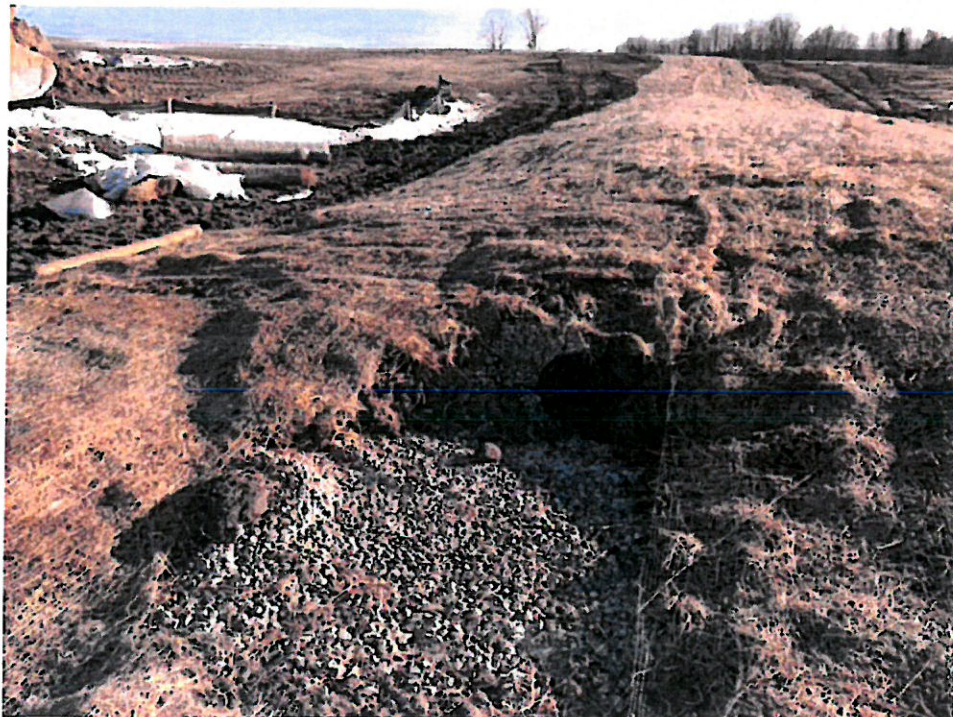
Photograph No. 15: Surface Berm and Swale Construction – Matting Placement and Swale Outlet (1/20/15)
