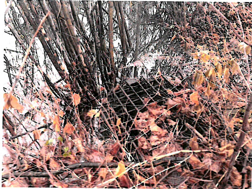
Photograph No. 6: Dinner Theatre storm water pond outlet structure (11/24/14)
