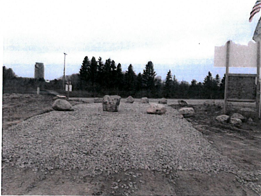
Photograph No. 10: M-72 access road facing north (12/04/14)
